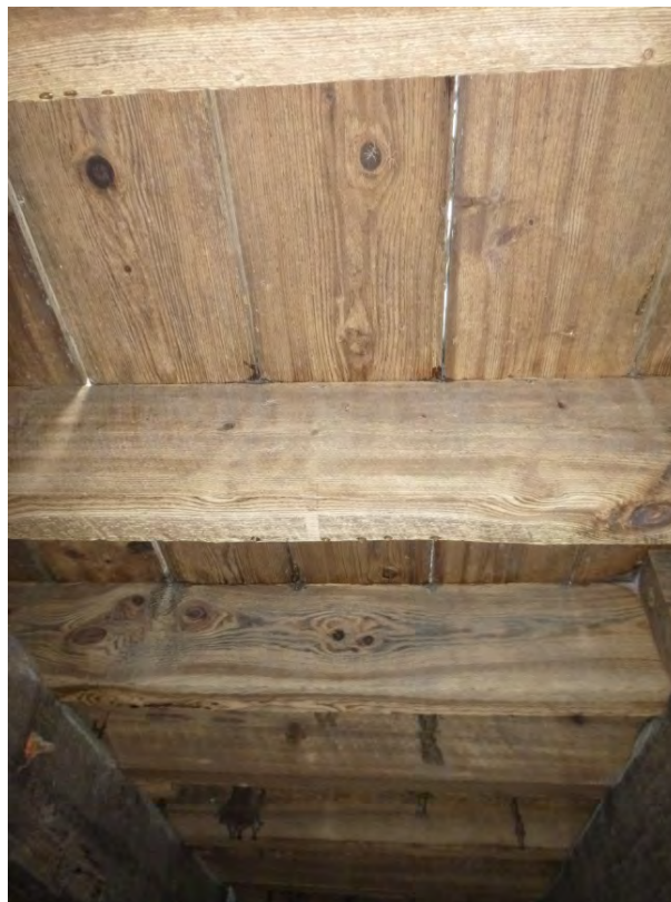
Photo 12 – Typical underside view of decking and stringers
