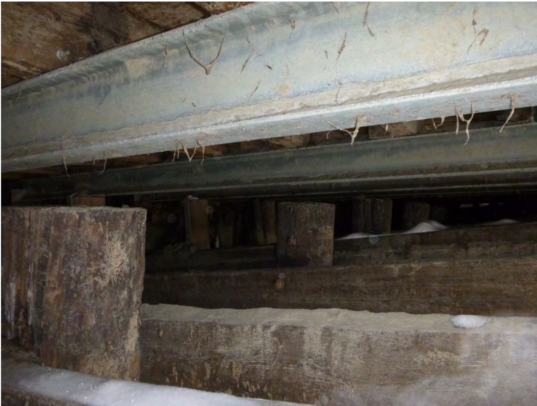
Photo 15 – Typical steel W200x27 girder
