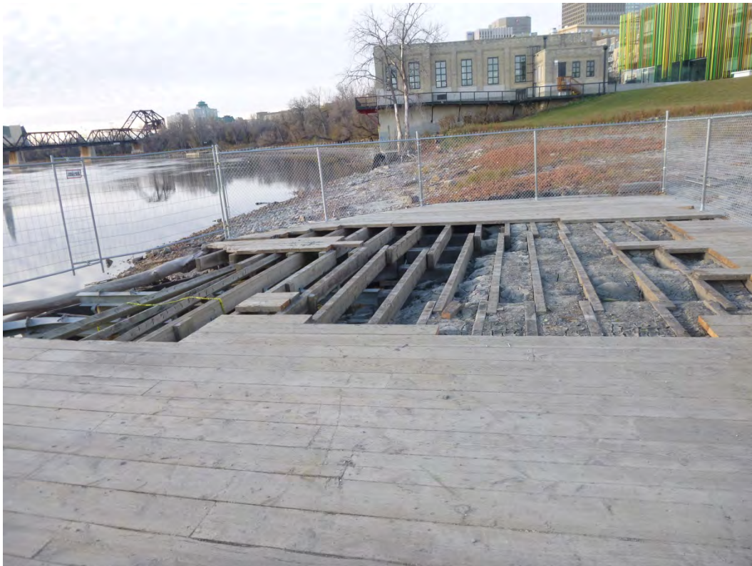
Photo 6 – South end of deck with exposed area for remedial works
