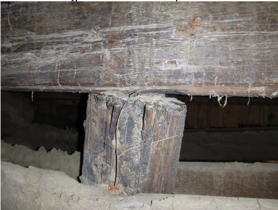
Photo 22 – Typical tilted pile support
