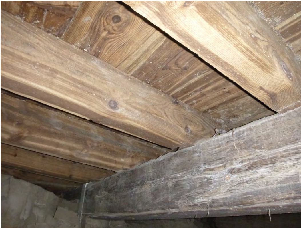
Photo 13 – Typical condition of timber pile cap beam
