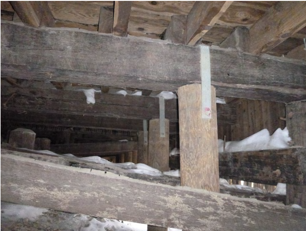
Photo 21 – Typical condition of remedial piles installed in 2004
